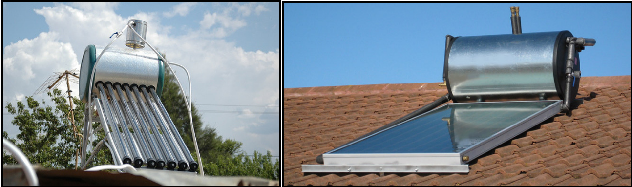
Figure 9-10: Typical solar geysers
