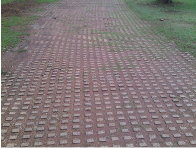
Figure 13: Paving proposed at Goegap Nature Reserve
