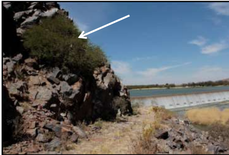
Figure 31 | The Boegoeberg weir with DWA access track and koppie on the east side. The small green tree amongst the rocks is Boscia albitrunca (Source: D.McDonald 2013).
