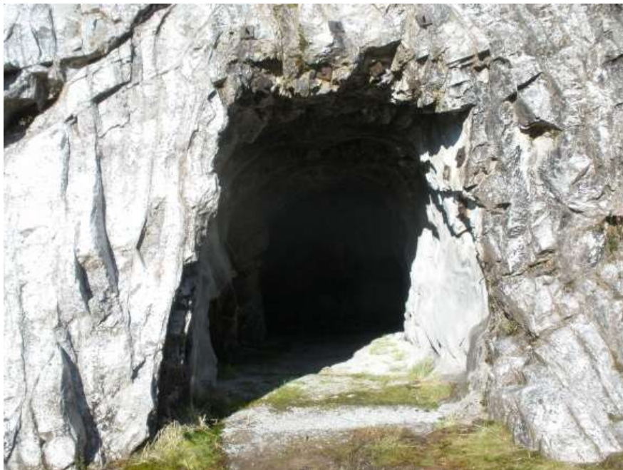
Figure 11 | Example of a Tunnel (Source: Entura)
