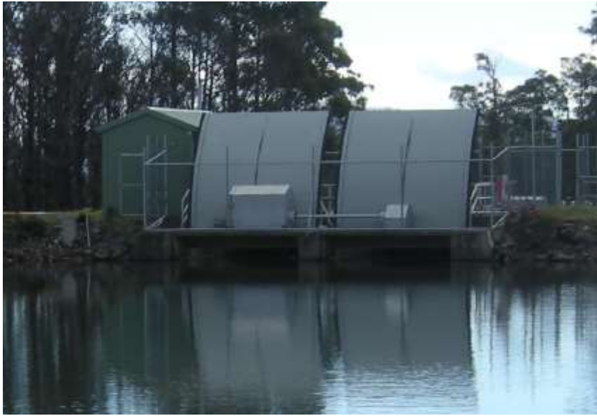
Figure 8 | Example of a similar intake structure with trash racks and cleaner (Source: Entura).
