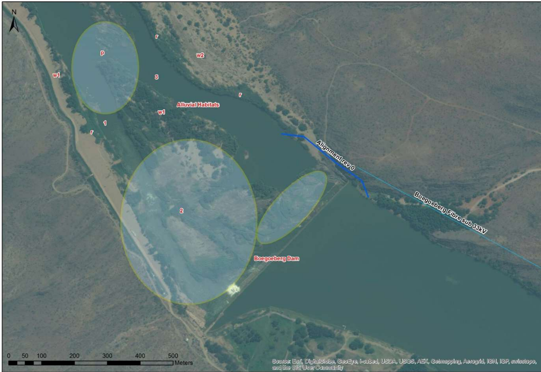
Figure 34 | Aerial view of the site to be impacted by the proposed development, showing 3 channels that comprise the main Orange River downstream of the dam wall, and the proposed alignment of the hydro scheme (dark blue line).
