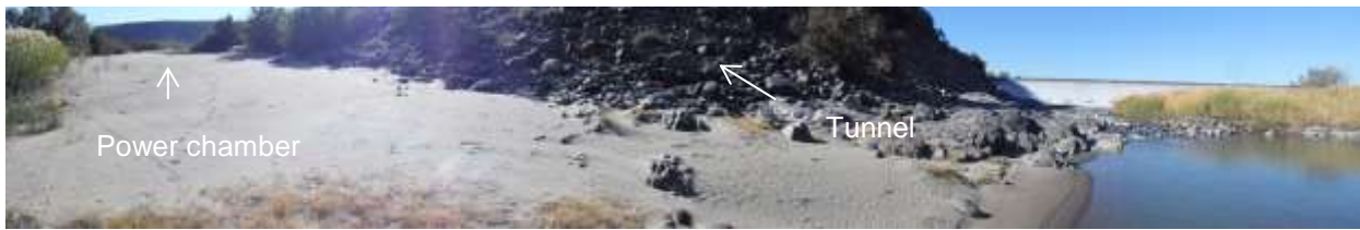
Figure 52 | View of the site where the power chamber is proposed. The weir can be seen in to the right of the photo. The canal would be tunnelled through the koppies.
