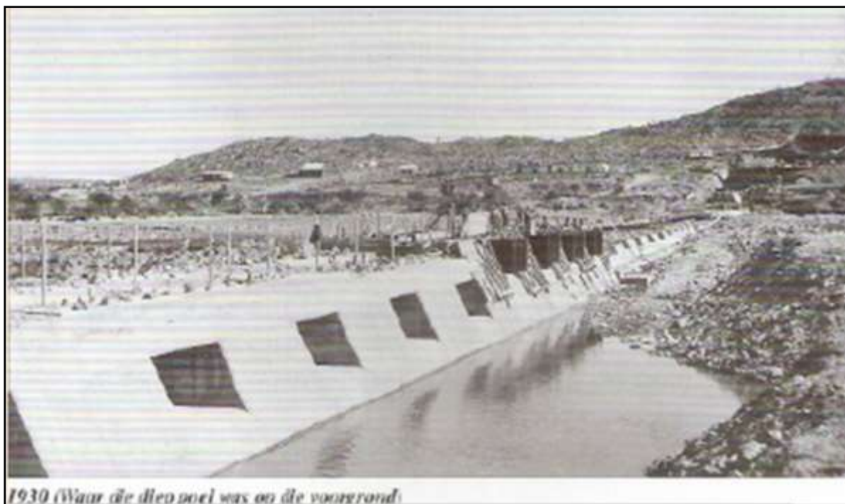
Figure 49 | Boegoeberg Weir during construction in 1930. Source: www.boegoebergcoroute.co.za .
