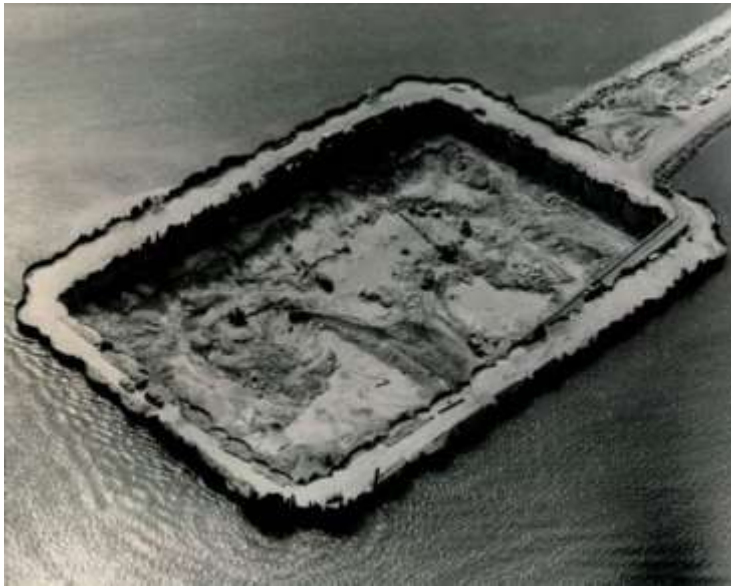
Figure 5 | Example of a coffer dam (Source: Cofferdam http://www.whalingcity.net/picture_hurricane_barrier.html )
