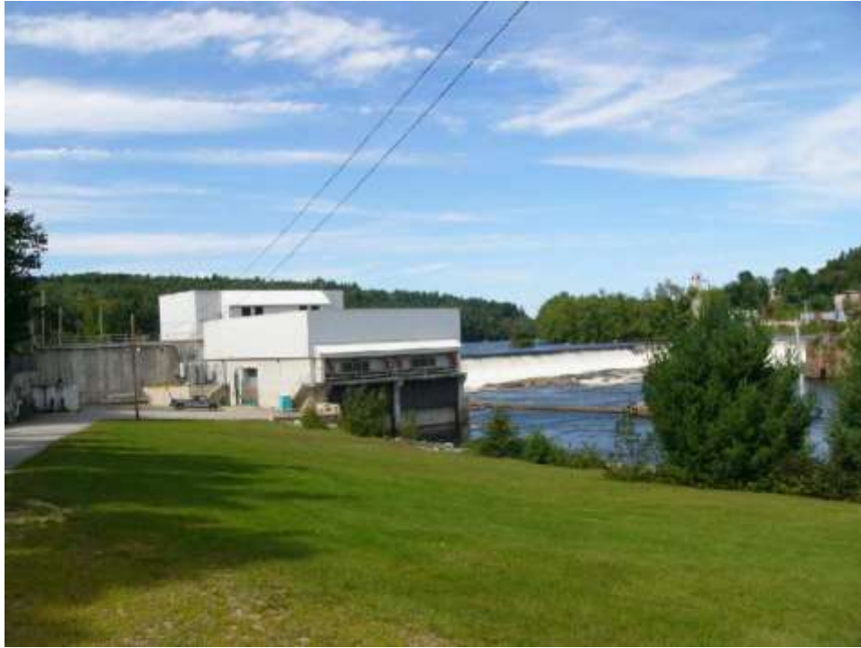
Figure 17| Example of a power chamber (Source: http://www.lowimpacthydro.org/ Accessed: 28 June 2013).
