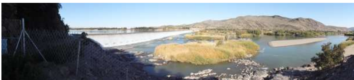
Figure 51 | View of the weir and area downstream of the weir close to where the canal and power chamber are proposed.
