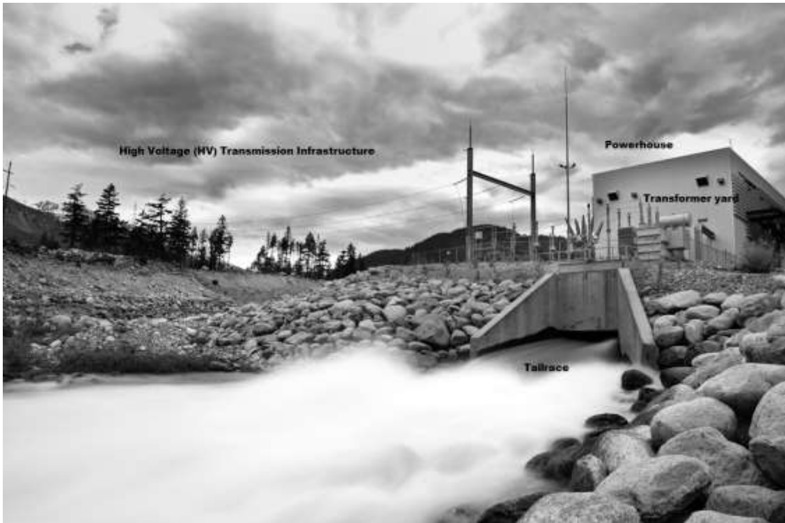
Figure 20 | Example of a power chamber and associated infrastructure. (source: http://www.photosensitive.com (Accessed: 28 June 2013)).
