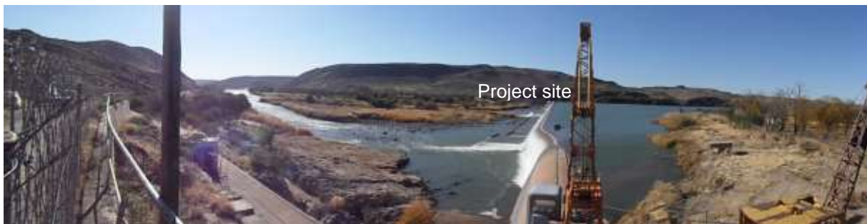
Figure 54 | View of the area downstream of the weir, with equipment for operation of the weir visible in the foreground, and the irrigation canal evident to the left of the photo.
