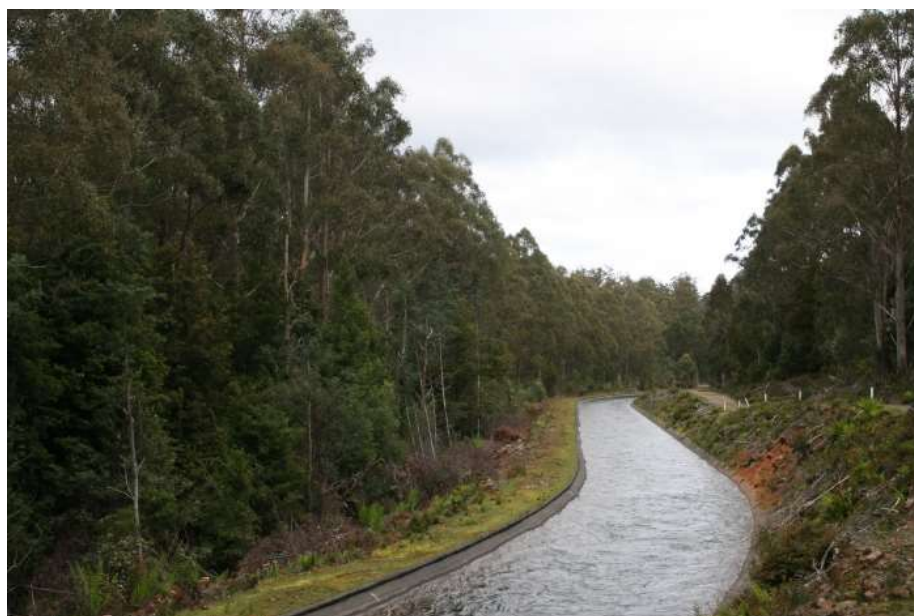
Figure 13 | Example of an open channel (Source: http://www.hydro.com.au/energy/our-power-stations/derwent (Accessed: 10 September 2013).
