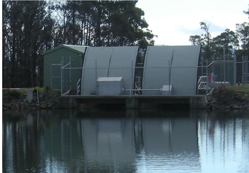
Figure 8 | Example of an intake structure with trash racks and cleaner (Source: Entura).
