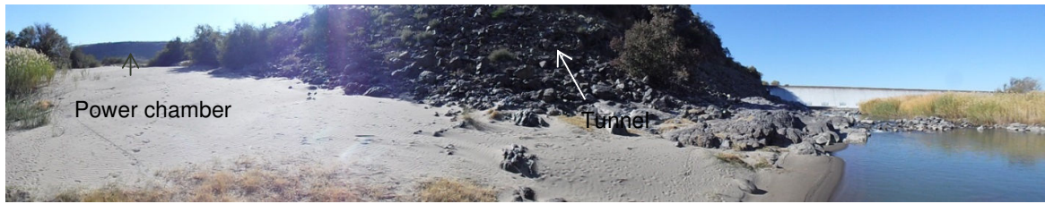
Figure 53 | View of the site where the power chamber is proposed. The weir can be seen to the right of the photo. The water conveyance infrastructure from the intake structure to the powerhouse would be tunnelled through the koppie.
