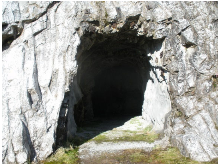
Figure 12 | Example of a tunnel (Source: Entura)
