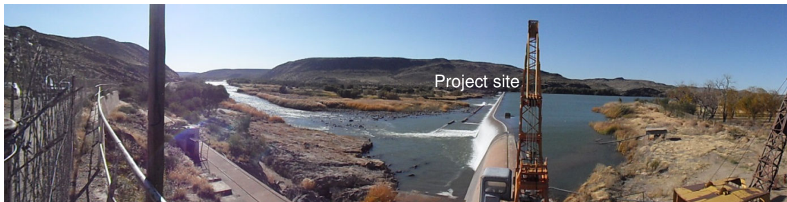
Figure 55 | View of the area downstream of the weir, with equipment for operation of the weir visible in the foreground, and the irrigation canal evident to the left of the photo.
