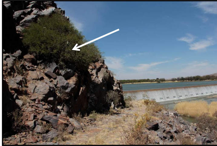
Figure 32 | The Boegoeberg weir with DWA access track and koppie on the east side. The small green tree amongst the rocks is Boscia albitrunca (Source: D. McDonald 2013)
