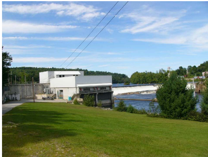
Figure 16| Example of a power chamber (Source: http://www.lowimpacthydro.org/ Accessed: 28 June 2013).
