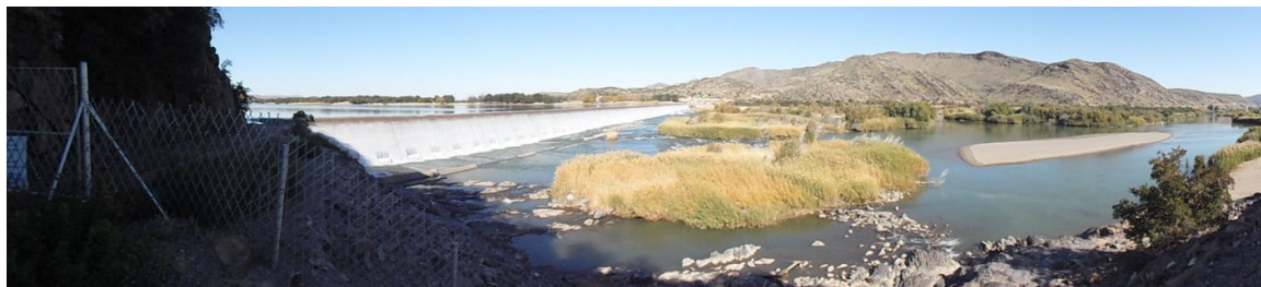
Figure 52 | View of the weir and area downstream of the weir close to where the water conveyance channel and power chamber are proposed
