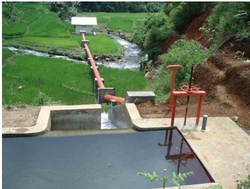
Figure 14 | Example of a small head pond (only applicable in the case of the canal alternative). (Source: energypedia.info (Accessed: 28 June 2013))
