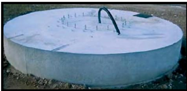
Figure 9-10: Foundation options for trackers
