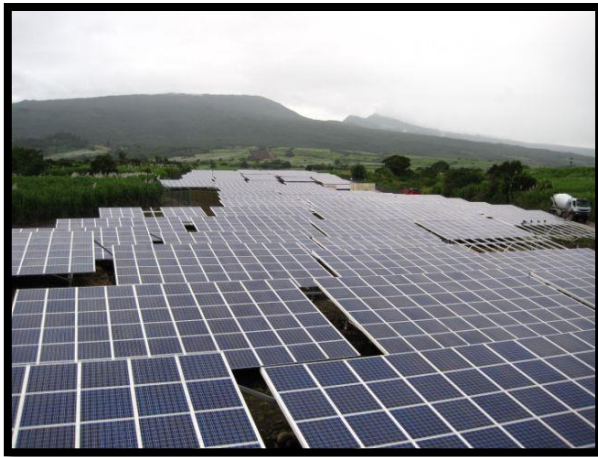
Figures 5-6: PV Solar Plant Consisting of Fixed Structures
