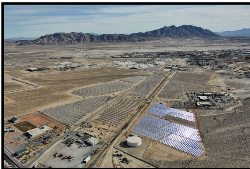
Figure 12: Nellis Air Force Base, Nevada, US (USAF, 2010)
