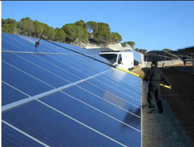
Figure 9: Cleaning PV panels
