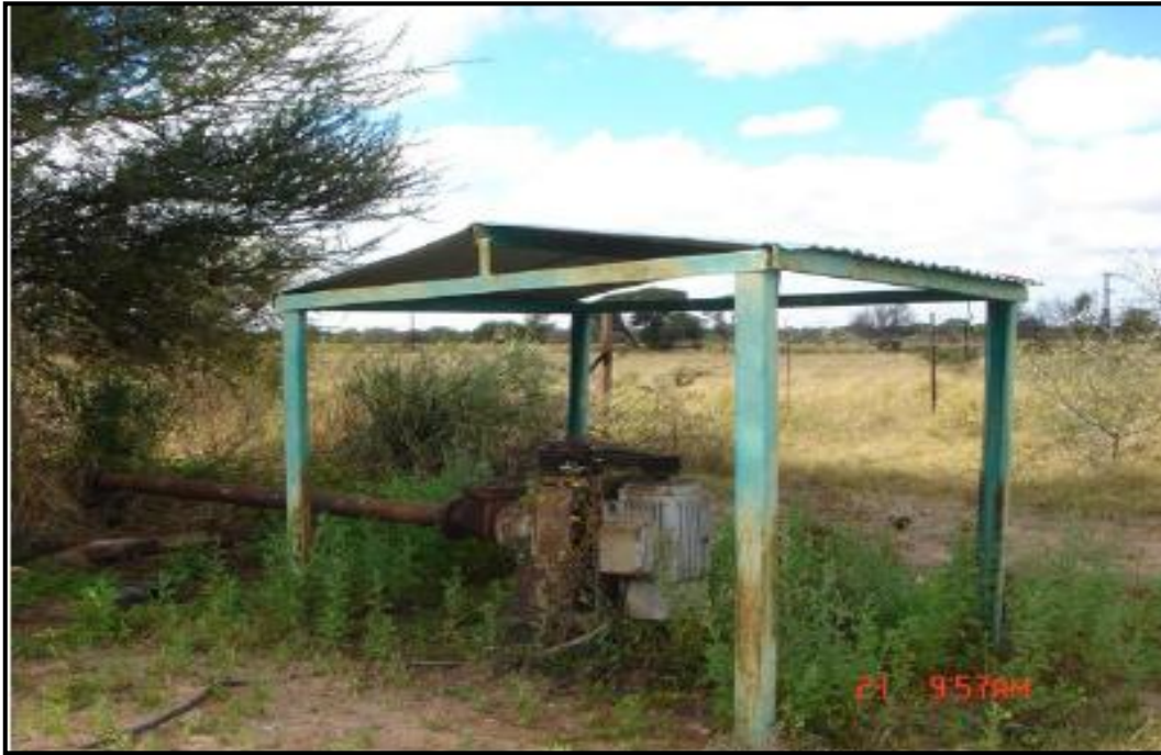
Figure 7: B-2 existing irrigation borehole (irrigates about 7ha)
