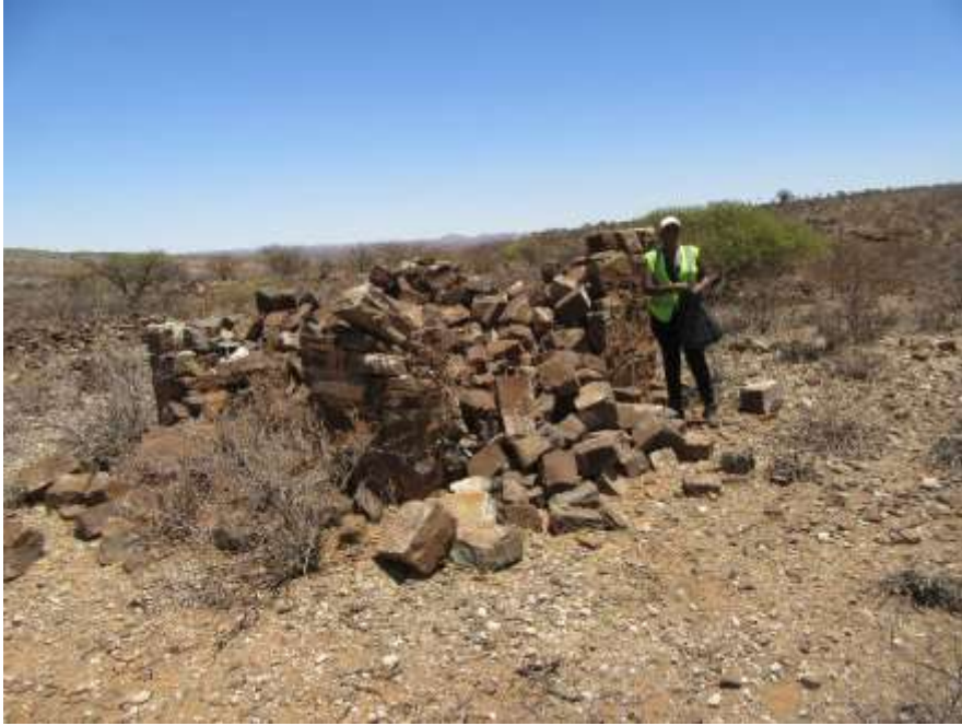
Figure 10: A small rectangular structure of dressed dolomite blocks, low rough walling to the south.
