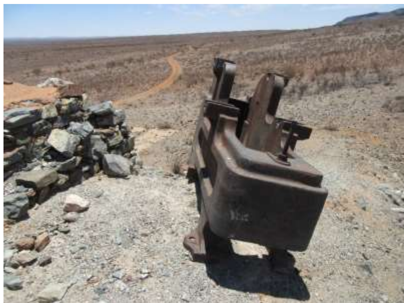
Figure 9a/b: derelict asbestos ore crushing/processing and loading bay of stonework and concrete.
