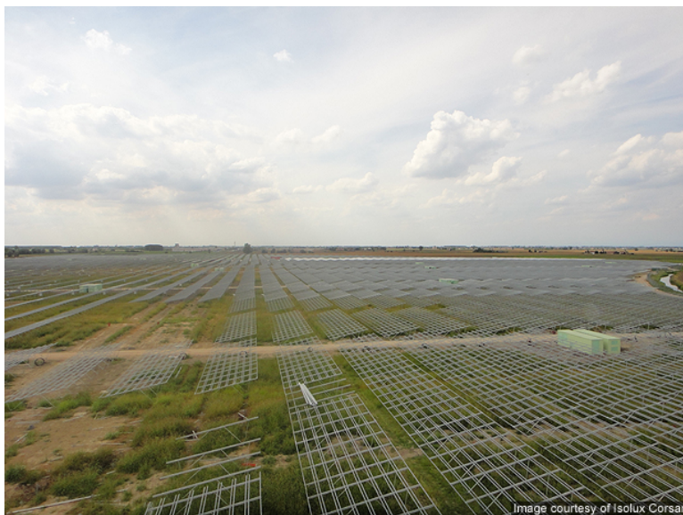
Figure 2.5: Example of erected steel mounting structures awaiting the installation of the PV panels (SunEdison Photovoltaic Power Plant, Rovigo, Italy)
