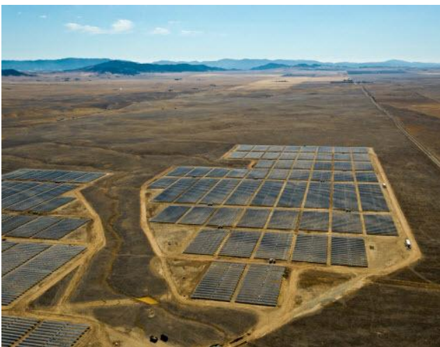
Figure 2 | Example of a PV facility in a landscape similar to Copperton
