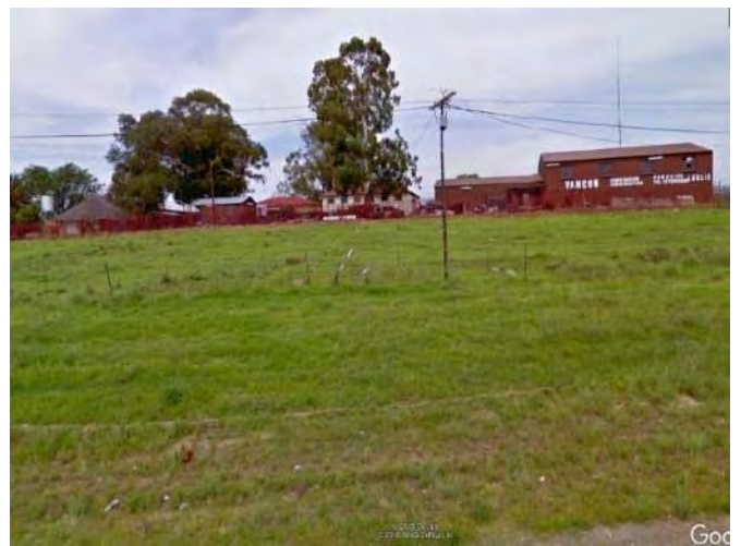
Business Buildings southeast of Leslie 1A surface infrastructure. Source Google Earth 2018
