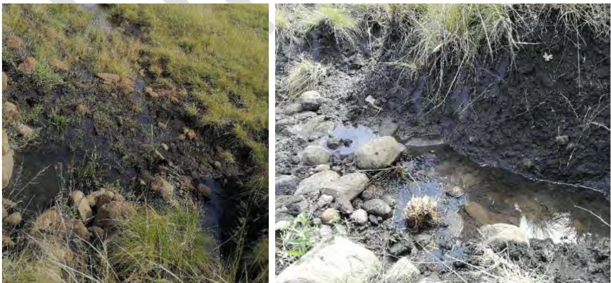
Figure 9-16: Typical erosion of soil seen on site. Here the profile has been subjected to erosion is a result of water movement over the land.
