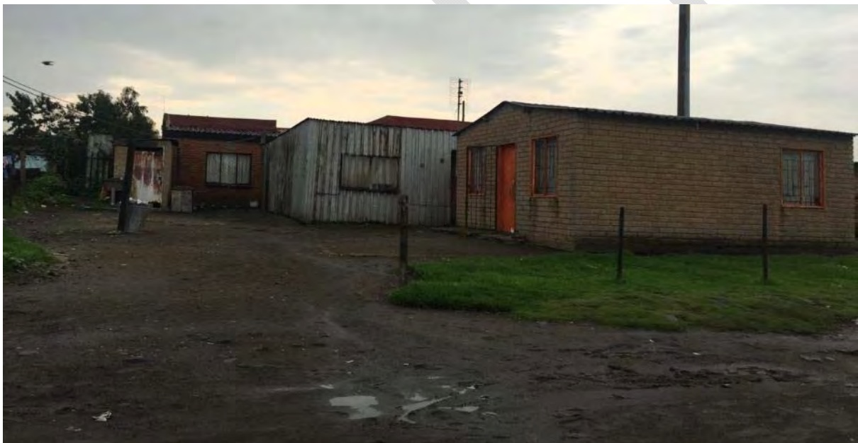
Figure 9-112: Housing structures in Leslie
