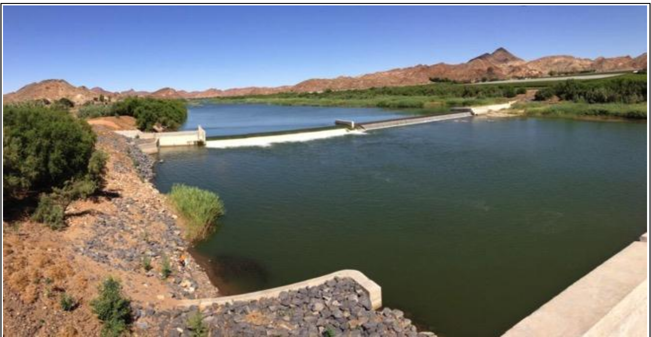
Plate 3.2: Blouputs hydrological gauging weir, Orange River, looking upstream
