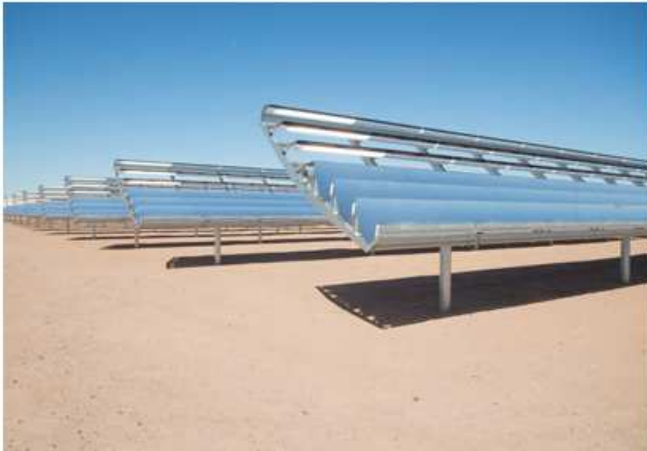
Figure 20: CPV panel using optics to concentrate the sunlight (image courtesy of Mulilo)
