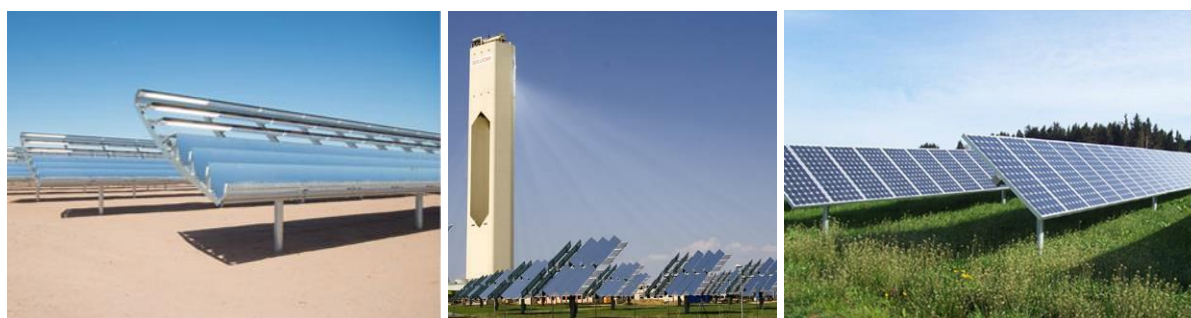
Figure 2.6 Photographs of CPV (left) 14 , CSP (middle) 15 and conventional PV (right) 16 technology
