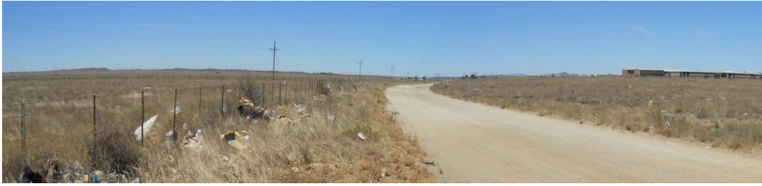
Fig 6.8 View along the north-south gravel road to the east of the townships along which the new transmission line servitude will run. A school can be seen on the right of the image
