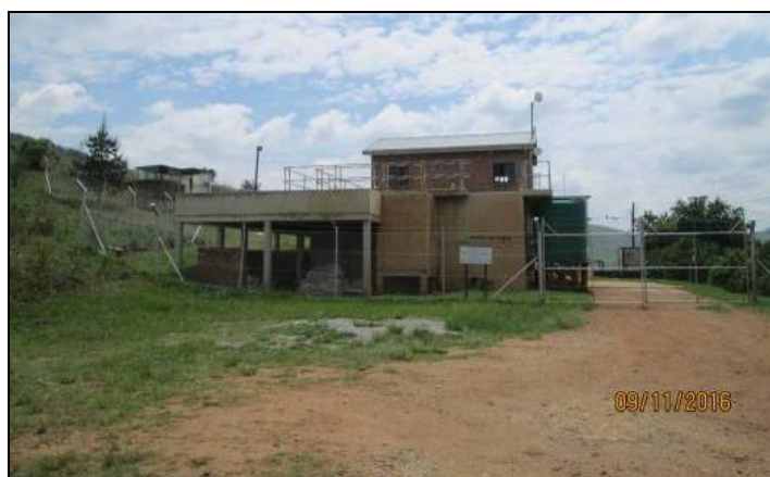
Photo 5.1: View of Amsterdam Water Treatment Works (WTW)
