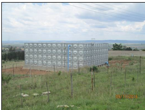
Photo 5.2: View of 2MI reservoir adjacent to the existing reservoirs at the Amsterdam WTW
