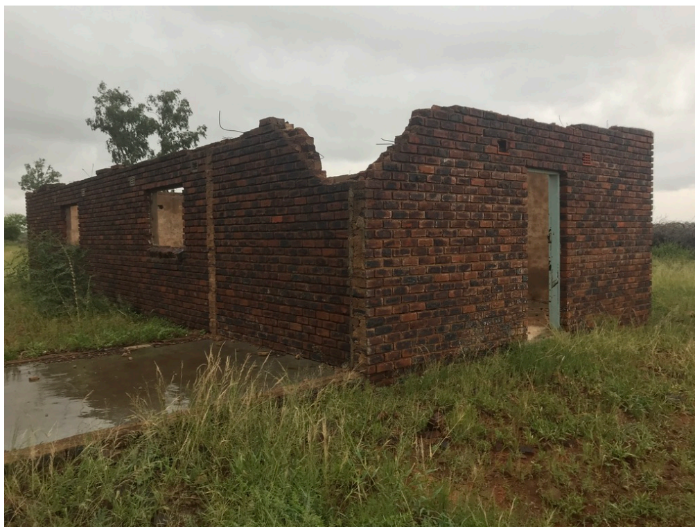
Photo 5: Close up of some buildings on the study site
