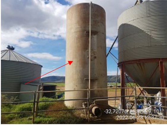
2 x Steel tanks storing effluent water for flushing of “standing apron”
