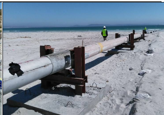
Figure 1-11 Typical Launchway across beach
