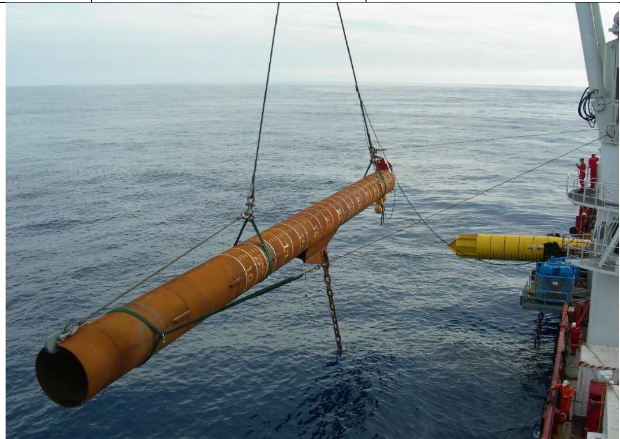
Typical anchor pile prior to being pitched and driven (source: Tekmar)
