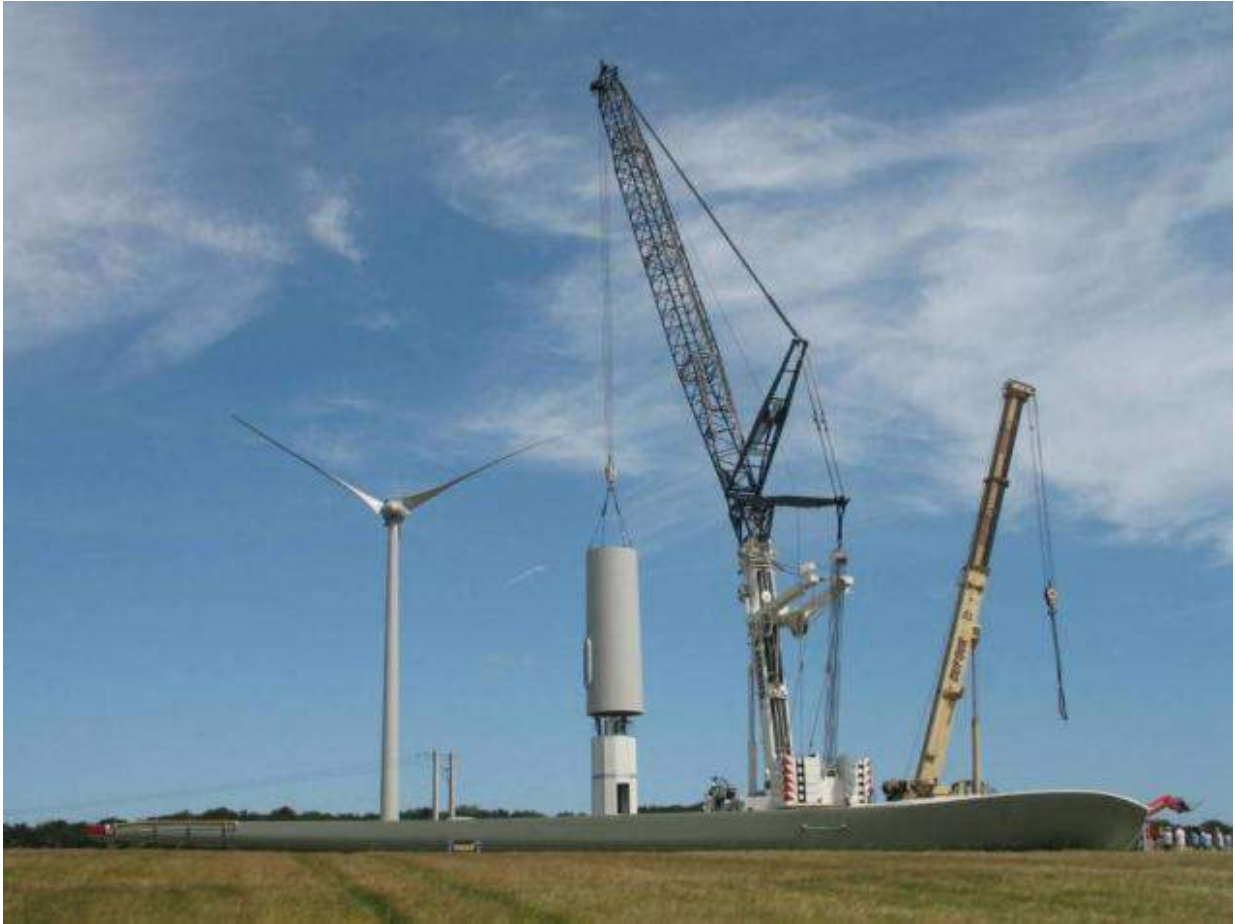
Figure 3: Assembly and erection of steel tower sections using cranes.
