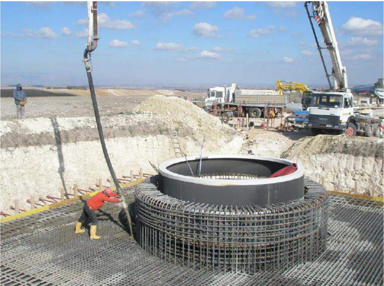
Plate 2-3: Concrete pouring of a turbine foundation – note the tower base collar in the foreground.
