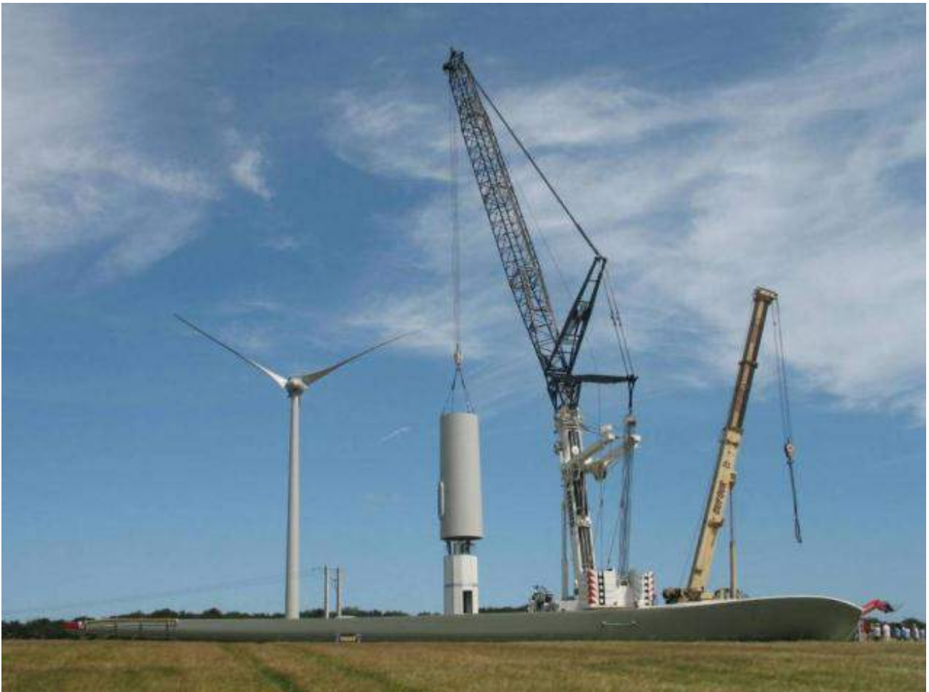
Plate 2-4: Assembly and erection of steel tower sections using cranes.
