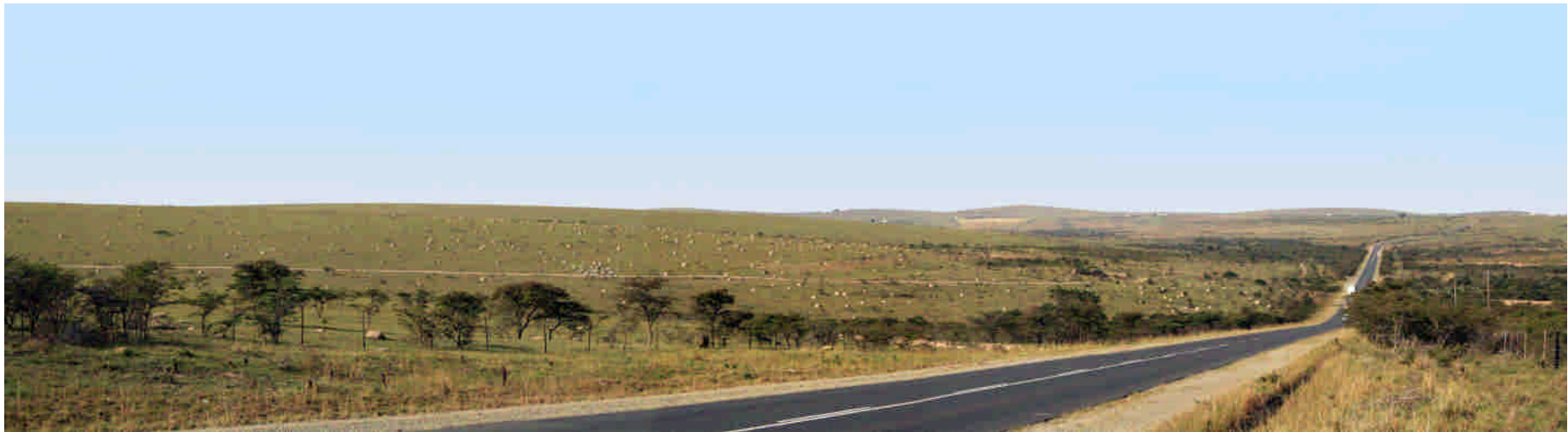
Figure 6.11: Pre-construction panoramic overview from Viewpoint 2
