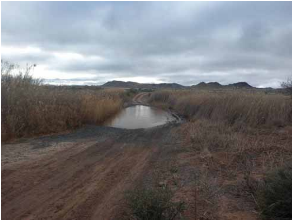
Existing road crossing a drainage area.
