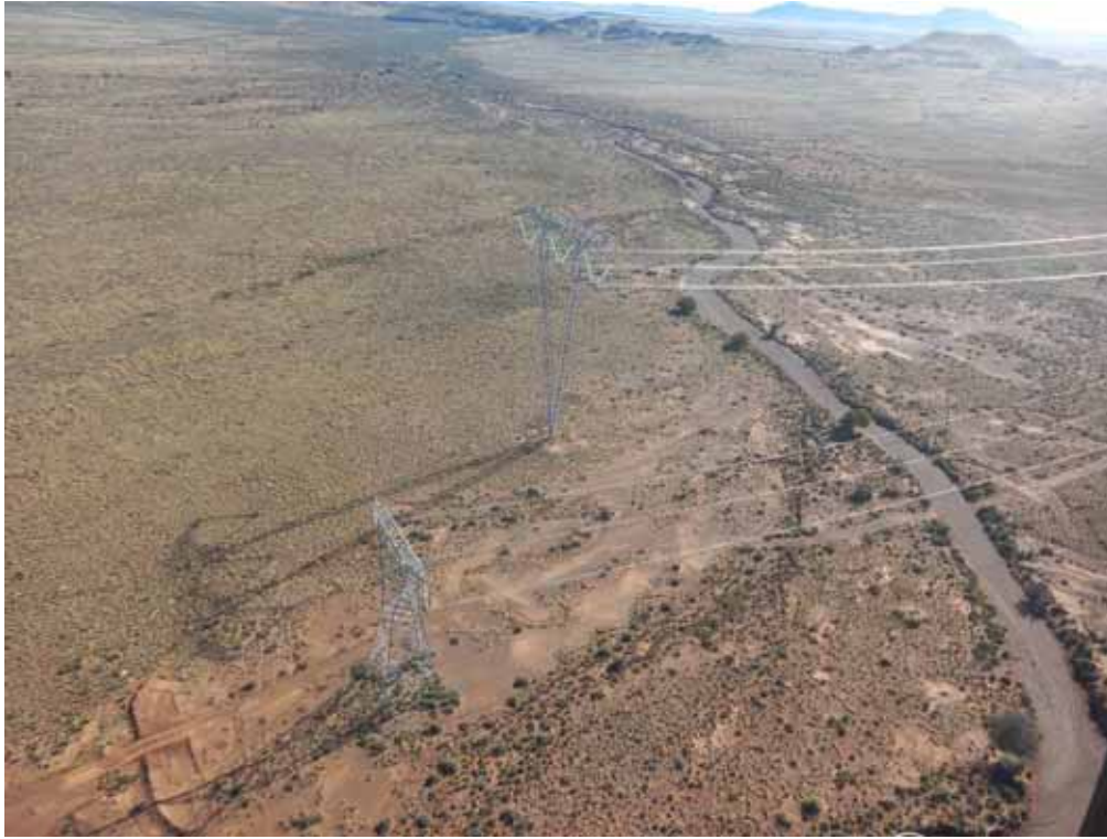
Plate 10: Pylons and access tracks in wide open floodplains near a main channel – exposed soils are at risk of surface wash and erosion, and stormwater management measures are important.
