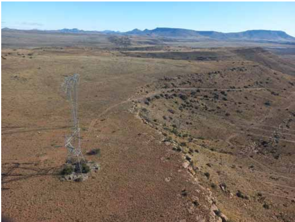
Plate 9: An existing pylon situated on a flat top, with an access track traversing a slope. The disturbance impact on soils seems to be limited to the pylon footprint and the access track with no obvious signs of erosion. The soils and rock in these areas are less prone to erosion, but care must be taken along access tracks to prevent channelized runoff and accelerated flow down slopes.
