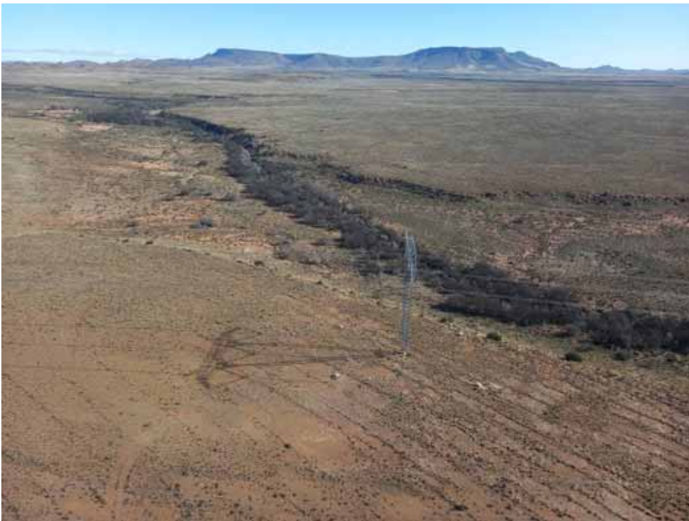
Plate 4: One of the existing gridlines on the eastern end of the Corridor, with a pylon placed to span the riparian area.
