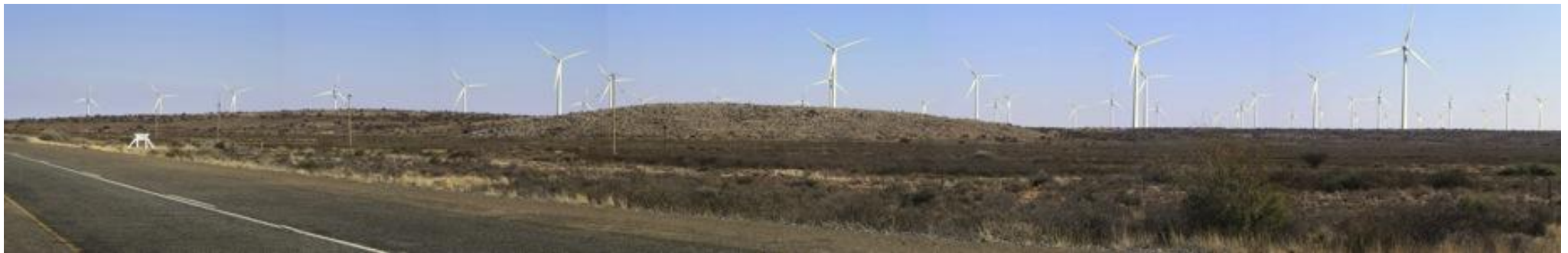
Figure 7.9b: Post construction panoramic overview from view point 1
