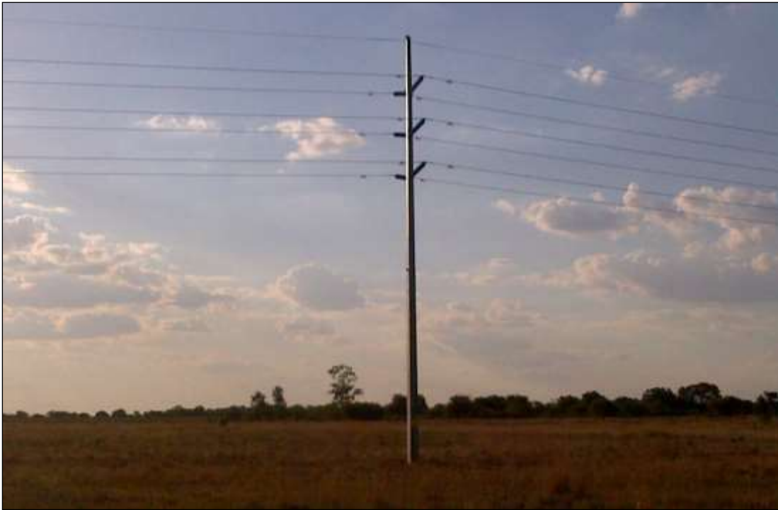
Figure 2: Steel monopole structure for a 132 kV power line (double circuit)
