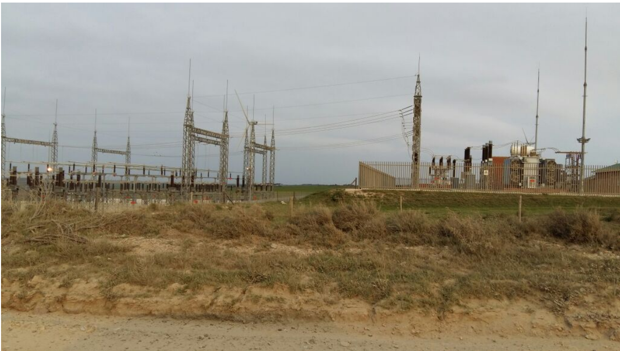
Figure 6.7: Substation / switching station
