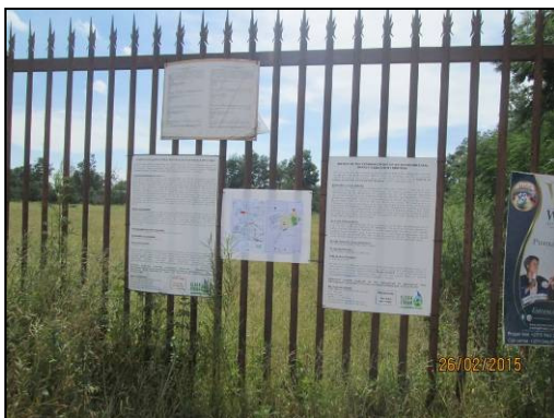
Photo 1: Onsite (western boundary) at the substation located adjacent to the Zaaihoek provincial road next to the MNS informal settlement.
