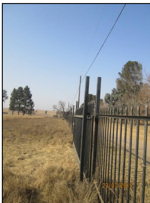
Photo 5.4: Eskom powerline and palisade fence on western boundary
