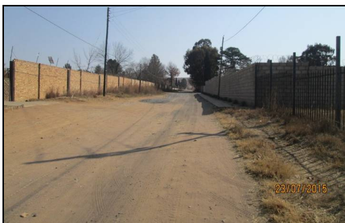
Photo 5.7: A view of Nyala Road looking towards the R555 provincial road
