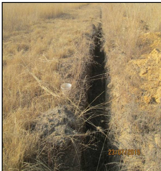
Photo 5.2: An open trench
