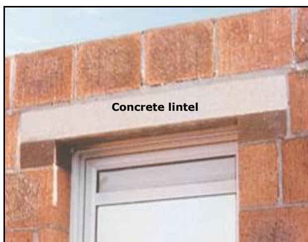
Photo 3.1: An example of a concrete lintel
