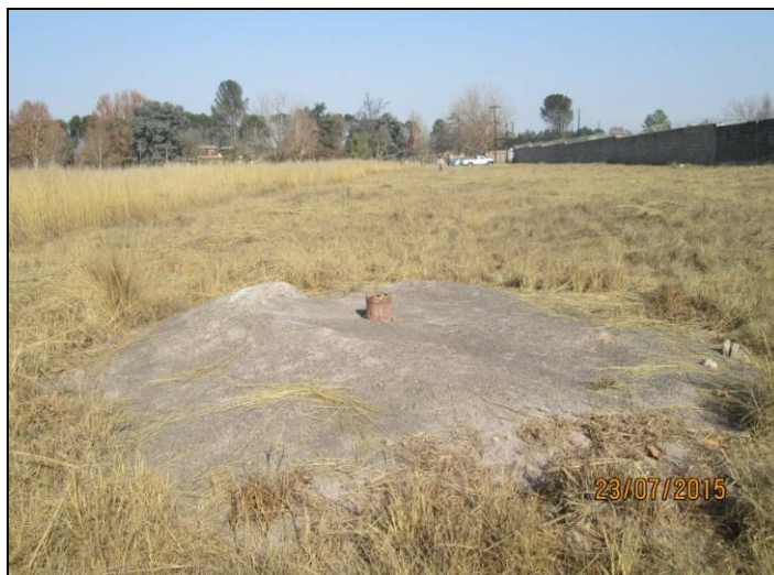
Photo 3.6: The newly drilled borehole
