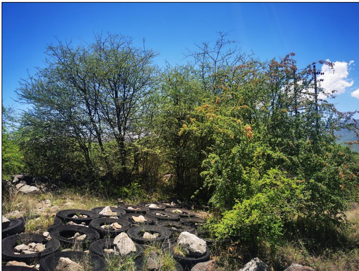
Figure 42: Illustration of tyres used for erosion control
