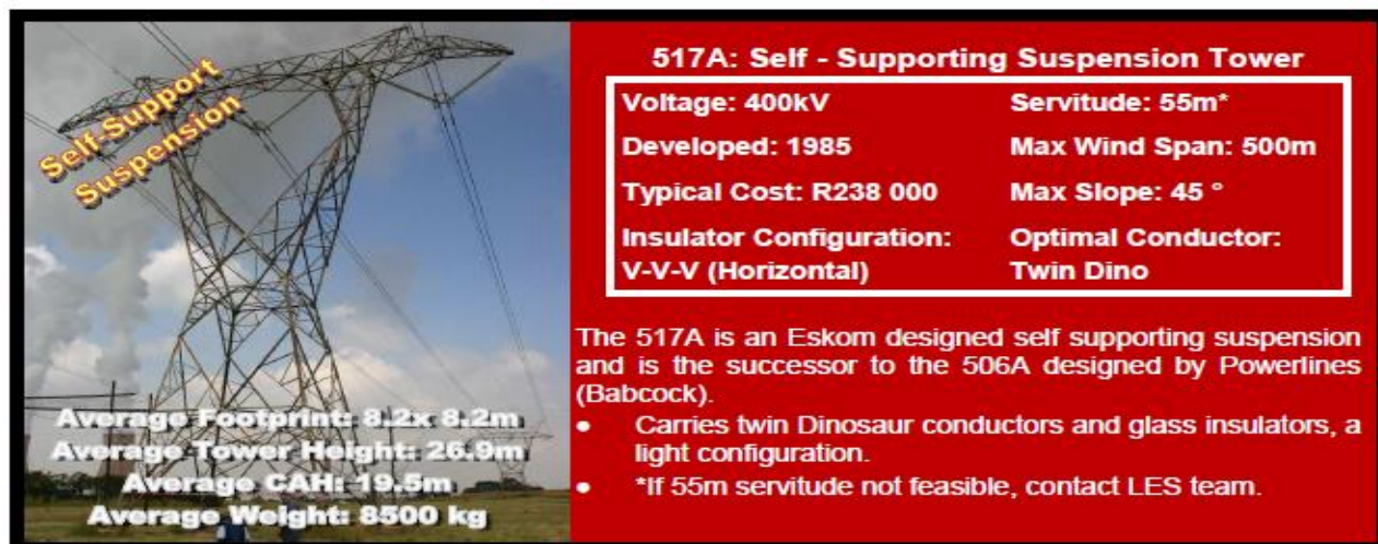
Figure 2-1: Example of a 517A self-supporting suspension tower 10
