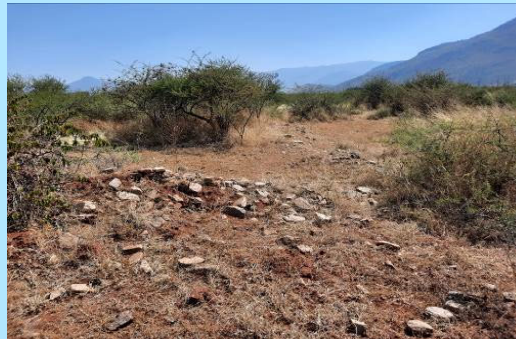
Figure 5-33: A series of broken-down structures and foundations
