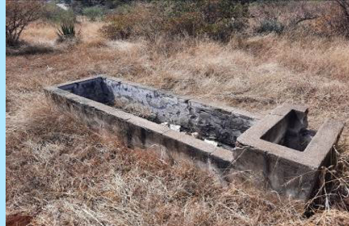
Figure 5-32: Cement water trough at Site 1-3
