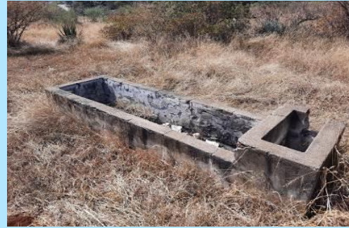
Figure 8-30: Cement water trough at Site 1-3
