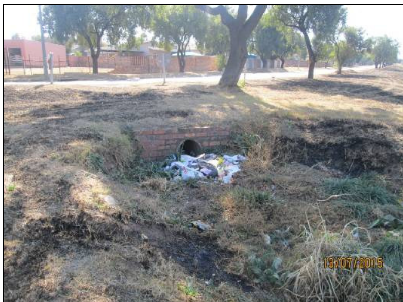
Photo 5.7: Kikuyu grass growing in the vicinity of the storm water culvert
