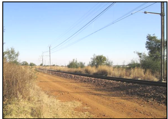
Photo 5.5: A view of the Transnet railway line and service road.
