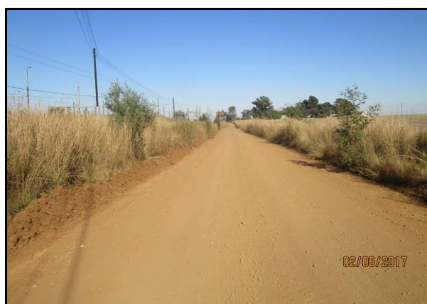
Photo 3.1: View of the existing access road adjacent to railway line
