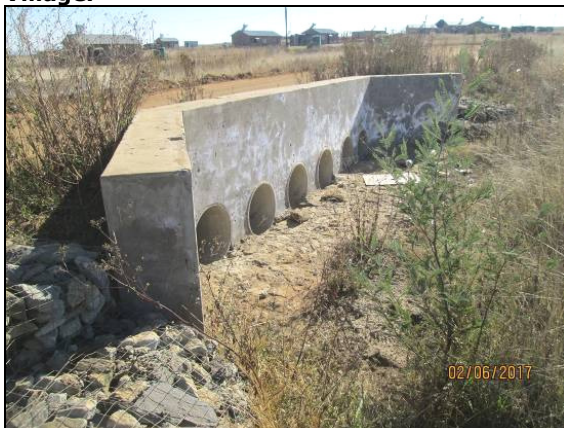
Photo 5.8: A view of the culvert located north of the site
