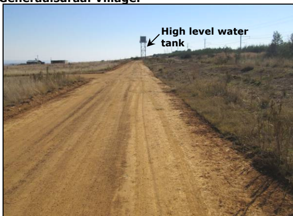
Photo 5.6: A view of the existing gravel road and high level water tank in Generaalsdraai Village.
