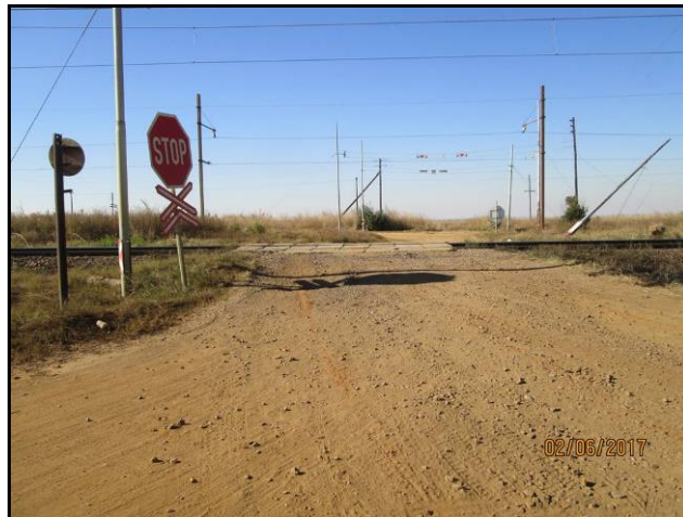
Photo 4.2: Existing level crossing across the railway line near the Afgri Silos
