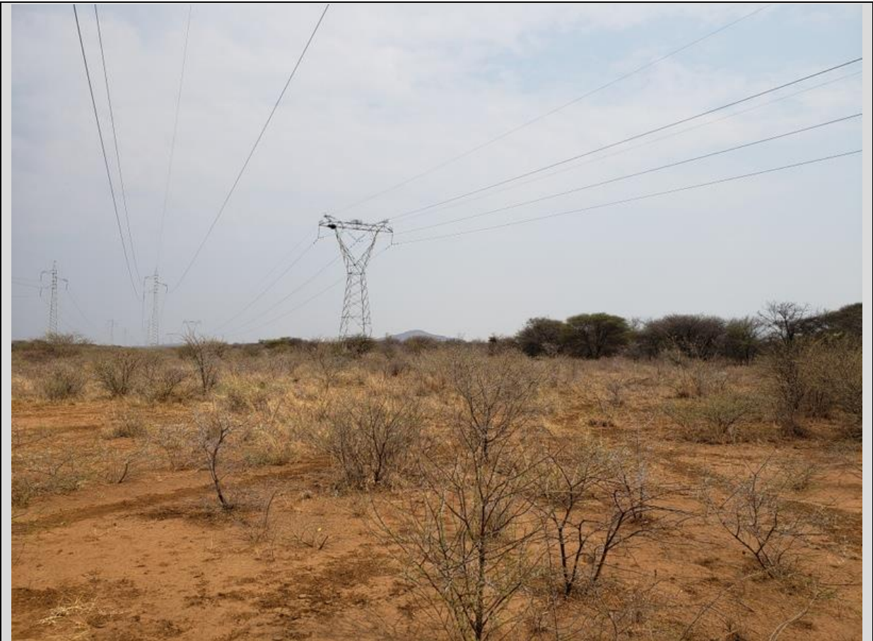
Plate 2: Eskom servitude traversing the site
