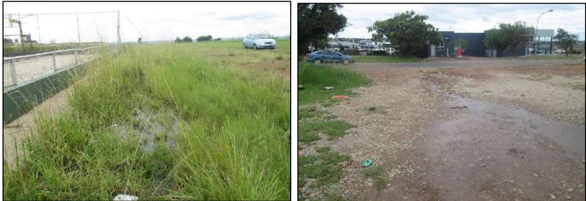
Photo 5.17: Storm water being diverted around the sports facility towards Nita Avenue
