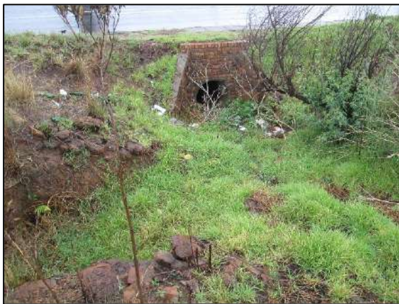
Photo 5.5: Storm water culvert under Mandela Drive Photo 5.6: Open sewer manhole
