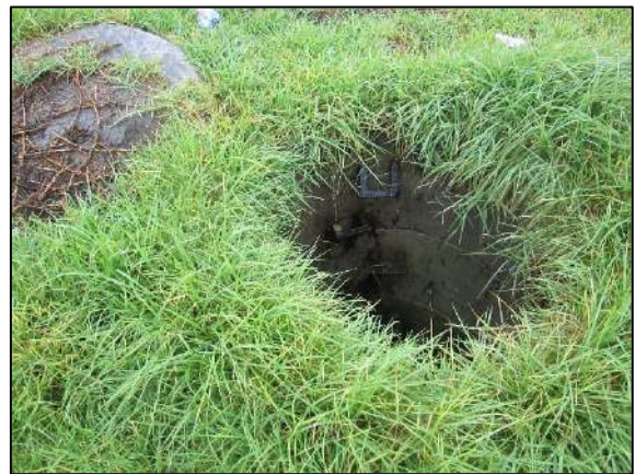
Photo 5.5: Storm water culvert under Mandela Drive Photo 5.6: Open sewer manhole
