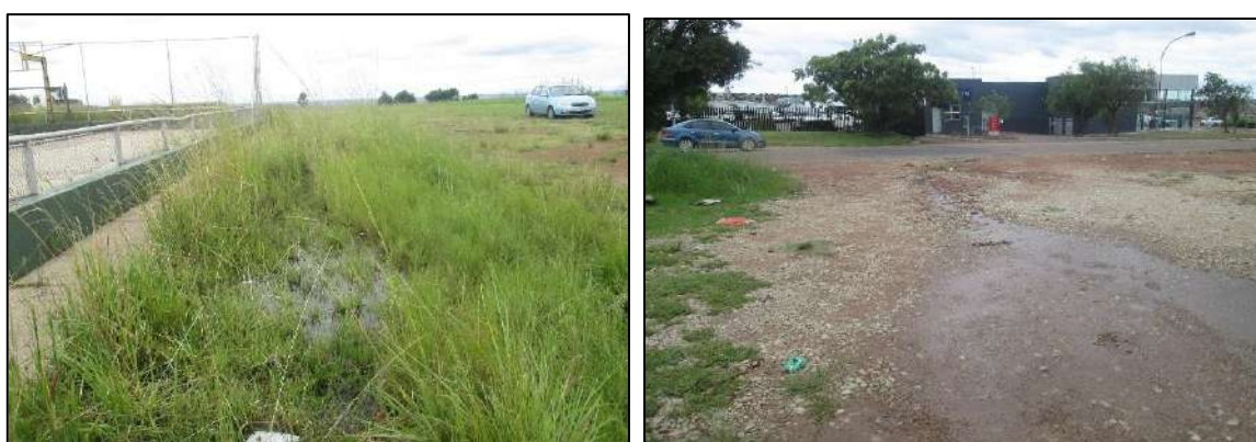
Photo 5.11: Storm water being diverted around the sports facility towards Nita Avenue
