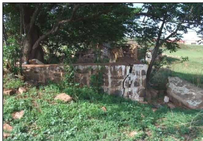
Photo 5.16: Remaining stone wall that may have been the foundation of a farm house
