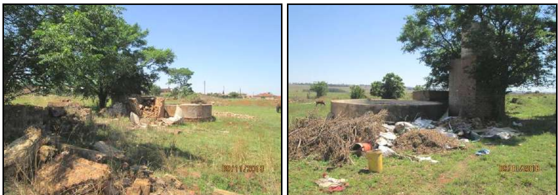
Photo 5.2: A view of the farmstead ruins in the southern portion of the site
