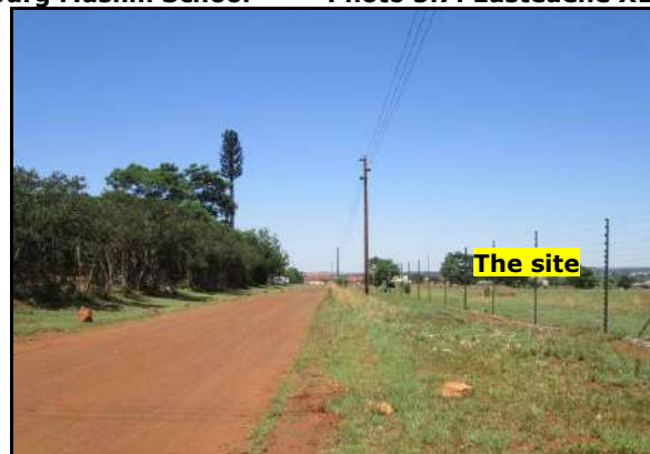
Photo 5.8: Right-of-Way gravel road and Eskom powerlines
