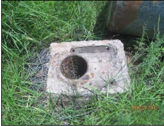
Photo 5.3: View of the old borehole
