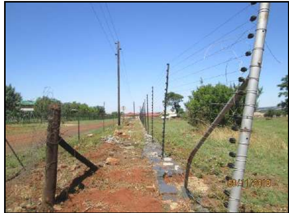
Photo 5.5: A view of the fence around the site
