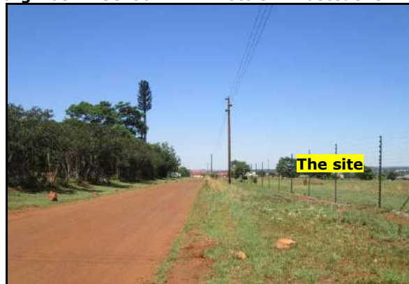
Photo 5.8: Right-of-Way gravel road and Eskom powerlines
