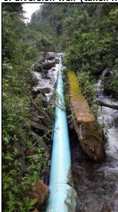
Photo 3.4: View of pipeline (taken from Kotze, 2015)
