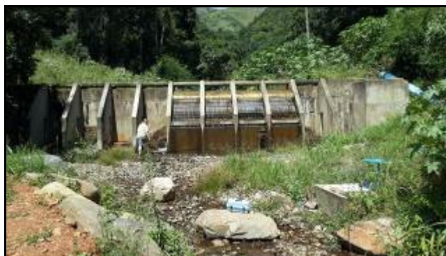
Photo 3.3: View of diversion weir (taken from Kotze, 2015)
