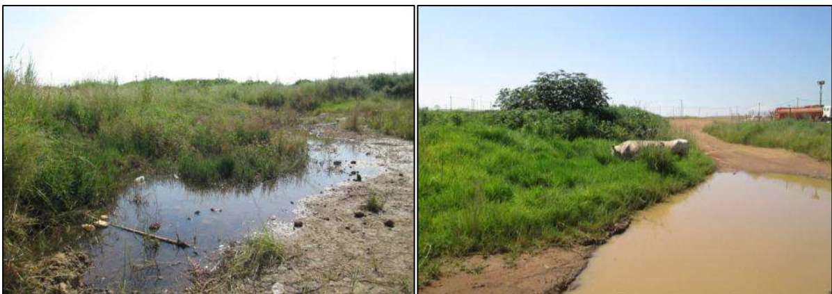
Photo 5.13: Ponding within the old borrow pit and along the gravel road
