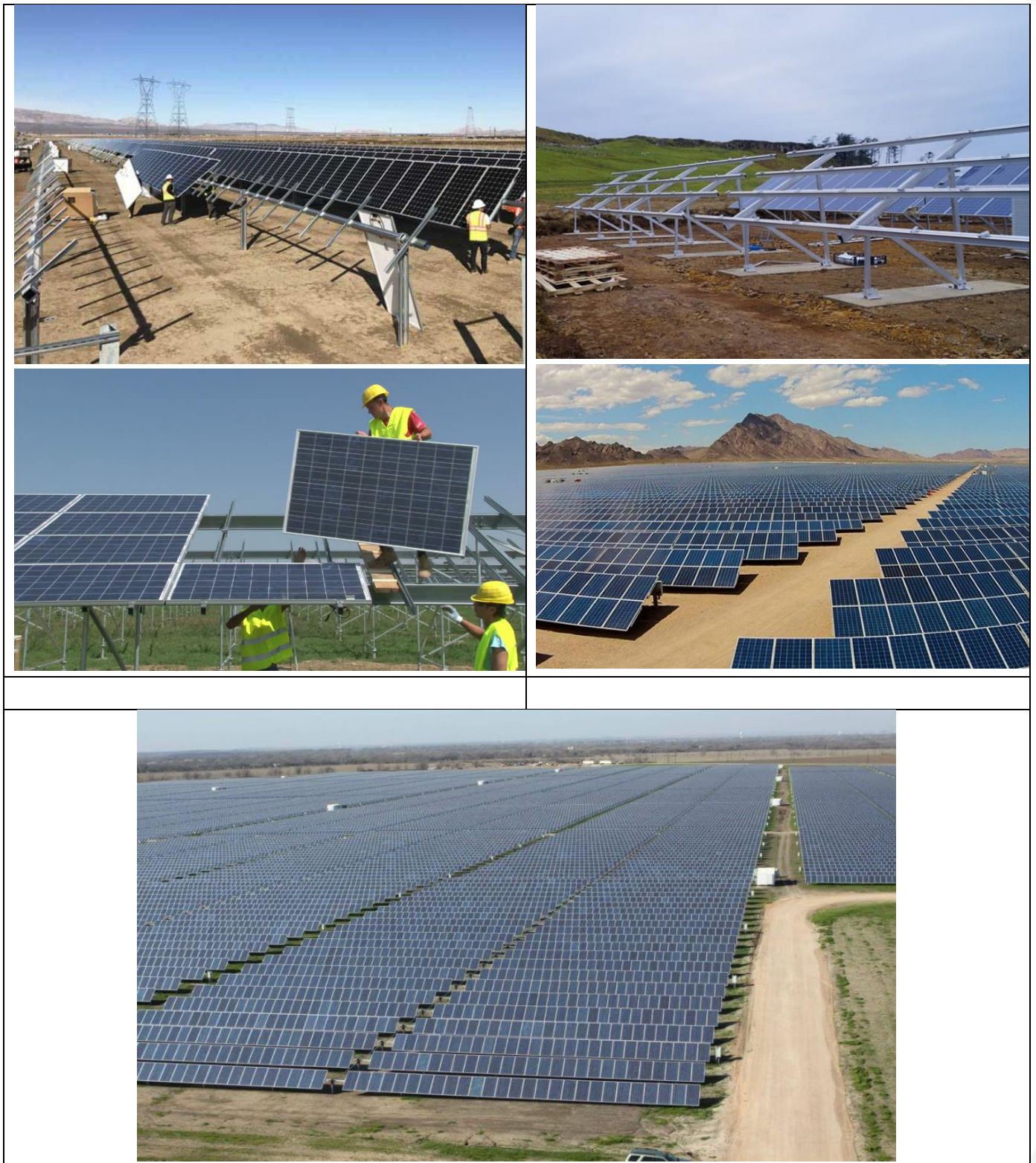
Figure 2.8: Photographs of the construction phase of a Solar Energy Facility similar to the Project (Source: https://medium.com/@solar.dao/how-to-build-pv-solar-plant-6c9f6a01020f ; https://www.shutterstock.com/video/clip-1028794-workers-mounting-panels-on-solar-power-plant-construction ; https://www.esi-africa.com/renewable-energy/kenya-construction-solar-farm-gets-green-light/ )
