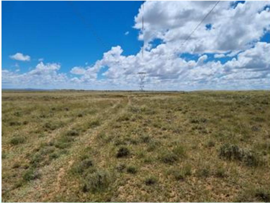
Photo 3. Existing 132kV ESKOM distribution line.
