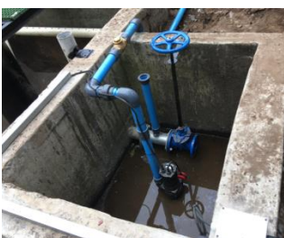
De-sludge chamber with de-sludge valve and Humus return pump
