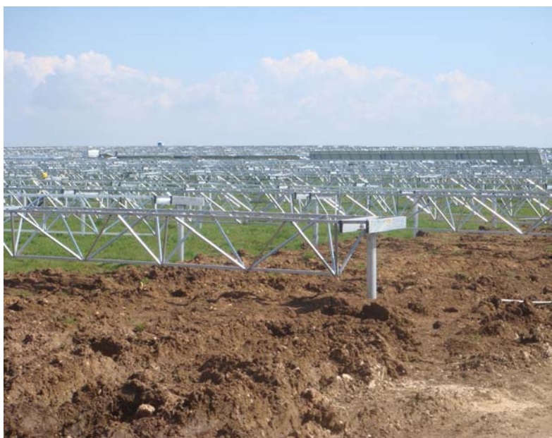
Figure 2.4: An example of site preparation activities that required the levelling some sections of the site.
