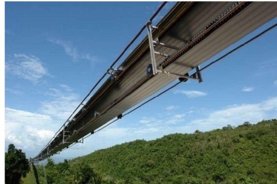
Figure 3. Typical RopeCon Section
