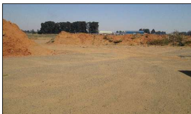
Photo 5.5: Recently cleared area with topsoil removed and stockpiled.
