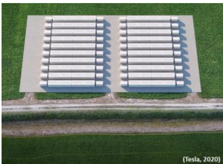
Figure 3.1: Conceptual design of a BESS indicating the use of modular containers
