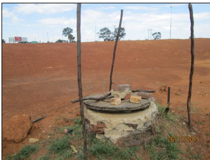
Figure 5.19: View of borehole
