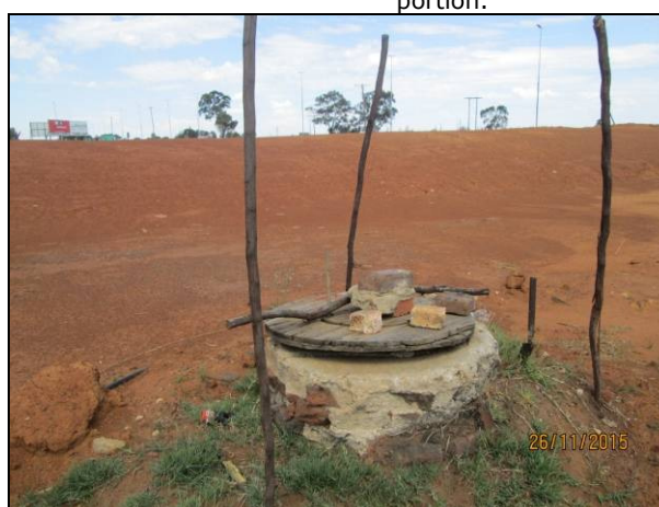
The borehole located adjacent to the levelled area.
