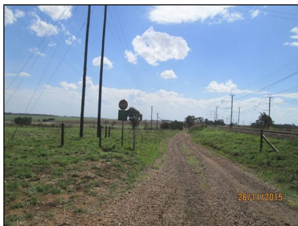
The Transnet railway line and servitude road.
