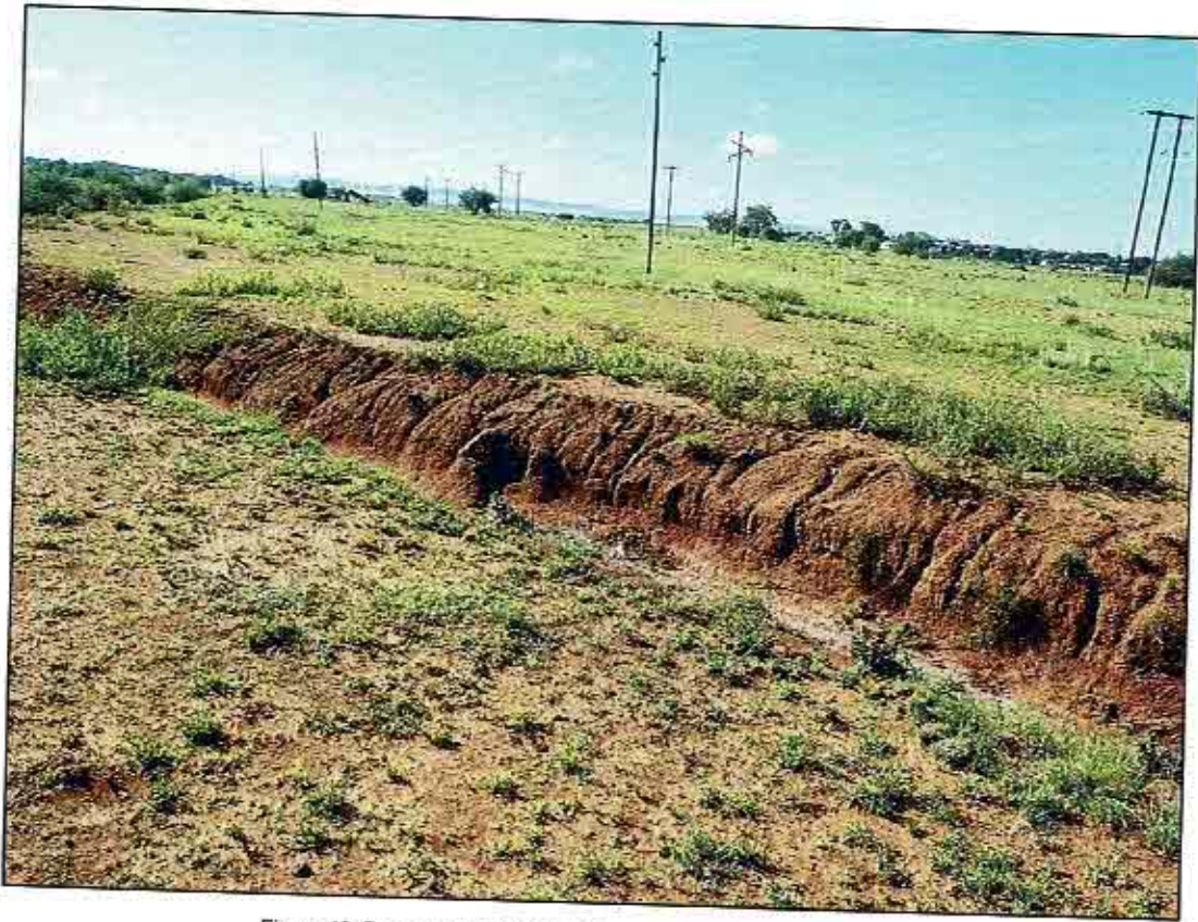
Figure 43. Drainage ditch at Area D
