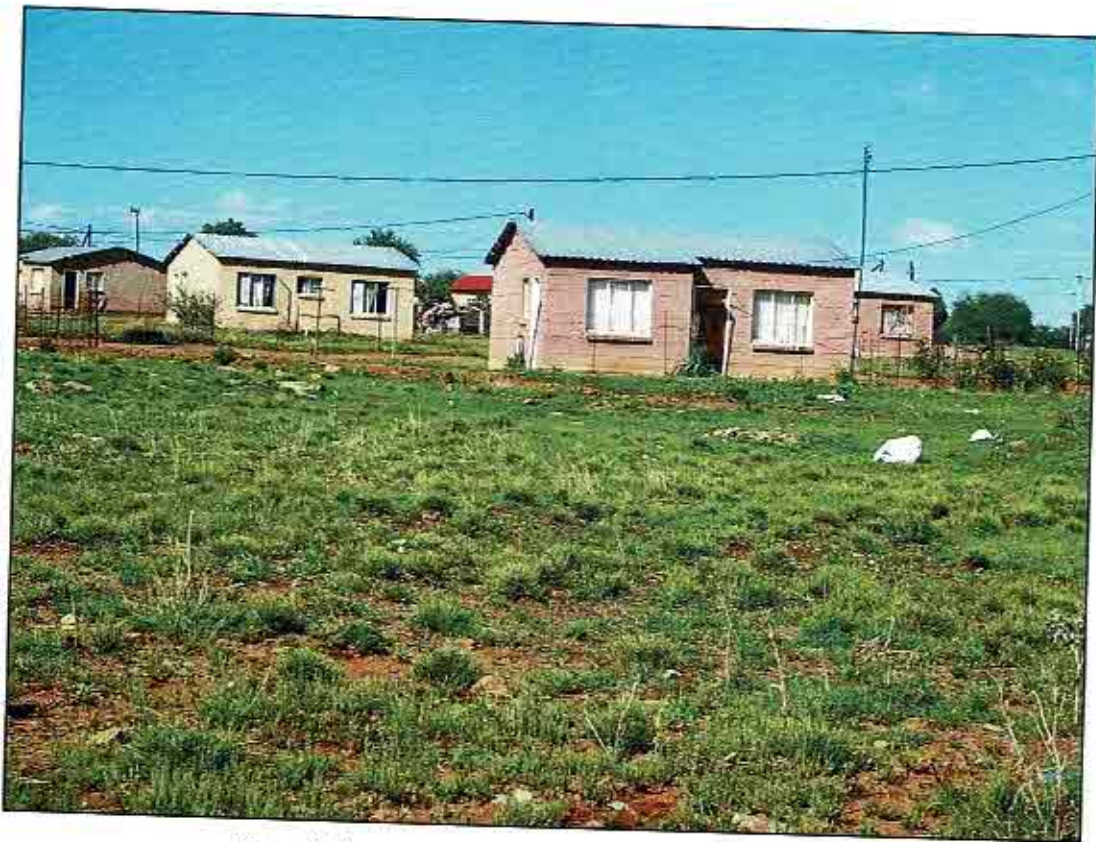
Figure 44. Houses at Ithumeleng
