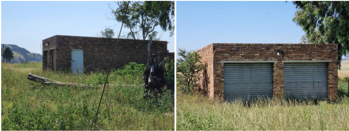
Figure 10.4-40 : Late 20 th century brick structure with metal roller doors.
