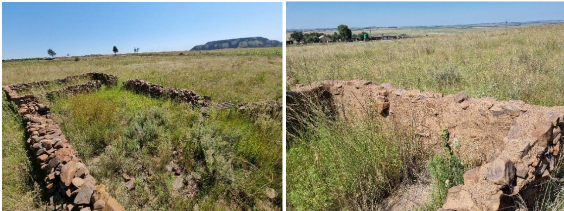
Figure 8-42 : UP-DRB-2529-02, (left) looking east over both rooms, and north (right) with cement plaster visible on inside of northern room.
