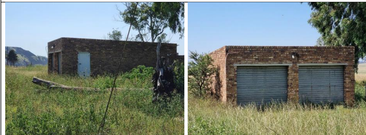
Figure 8-40 : Late 20 th century brick structure with metal roller doors.
