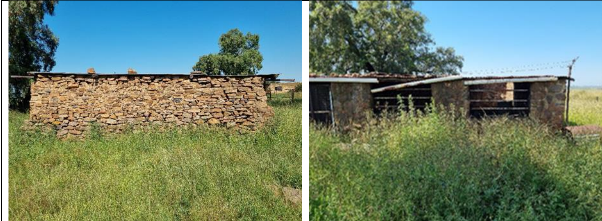
Figure 8-39: Likely storeroom and livestock/pen/chicken coop. South facing wall (left) and northwest corner (right).
