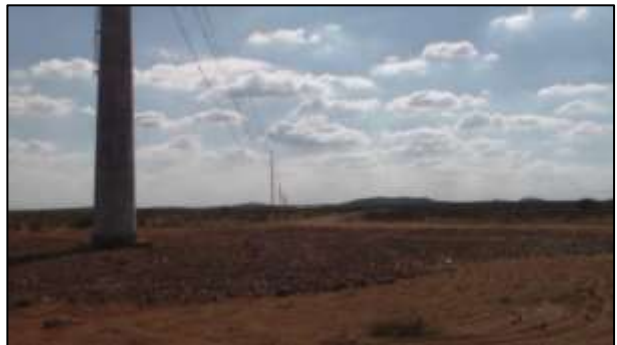
OBS 65 Pylon where access road begin (28/02/2020)
